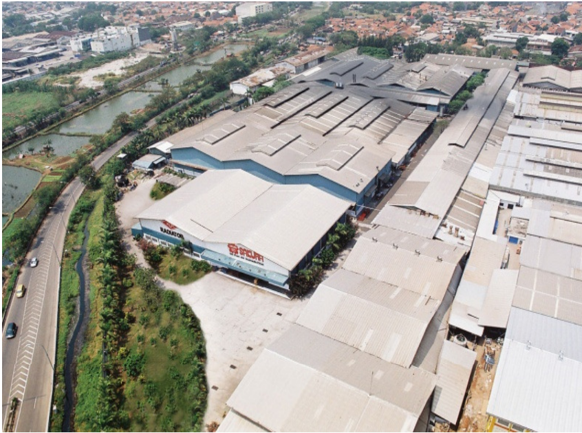
Kapuk Plant (Radiator Facilities)
